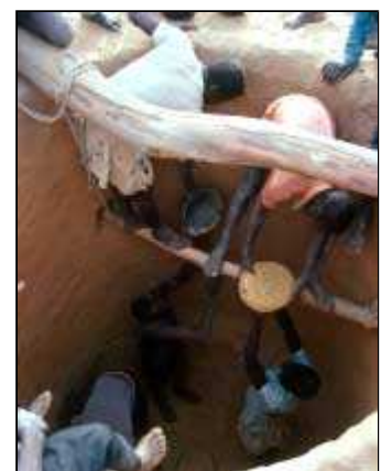
construction of a well
